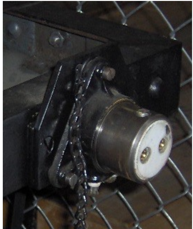
Stromstecker Aggregat (Foto 6)
